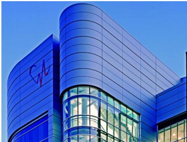
Figure 1: Office building with metal panel enclosure
